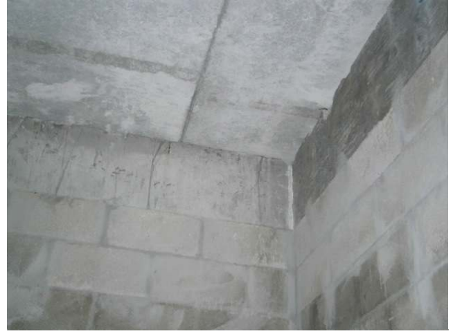
REINFORCED CONCRETE ROOF DECK ON REINFORCED CONCRETE WALLS
